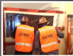
Local 67 Union Reps survey a containment area at a job site
