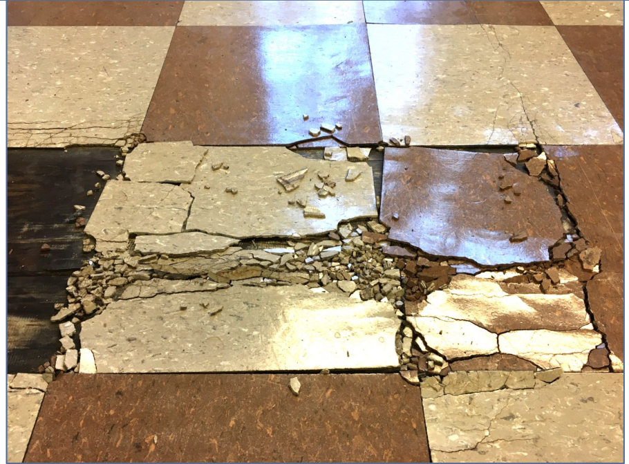
Photo of a floor tiles crumbling as a result of flooding.
