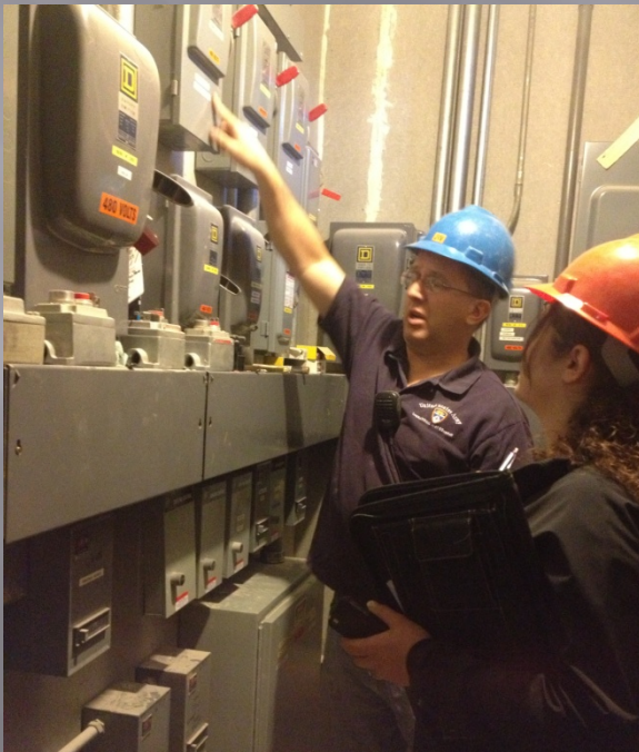
Electrical Room Inspection
